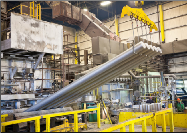
Figure 3. Pennex is among the many aluminum companies that have expanded secondary aluminum billet casting capacity.
